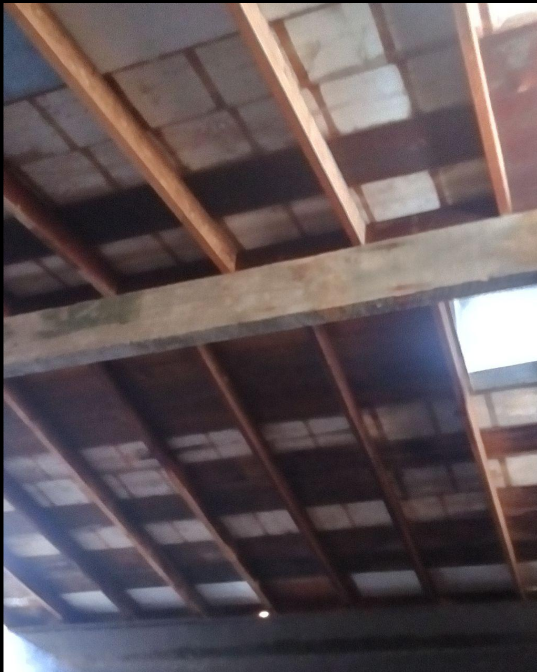
Tank #2 Inside Roof
