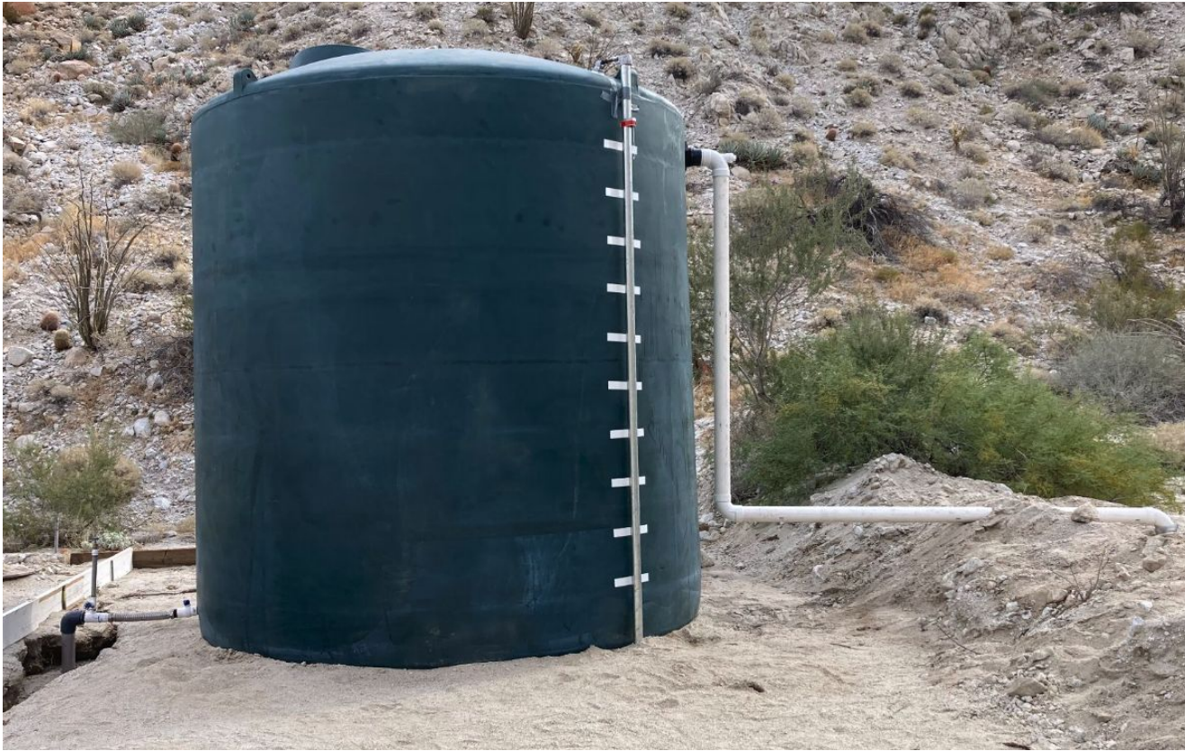
Tank #3 Approved for Operation January 5, 2024
