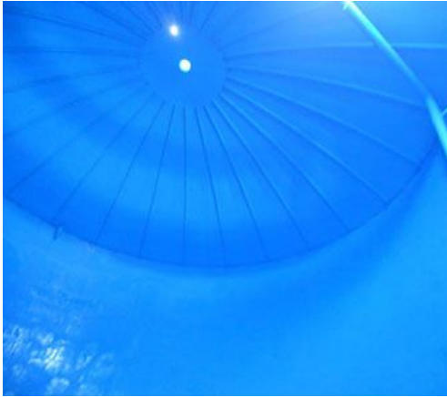
Steel Tank Liner
