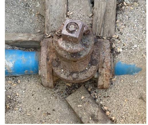
Replace Old Valves
