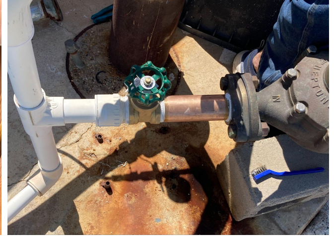
Gate Valve Upgrade for Mooney Pump
