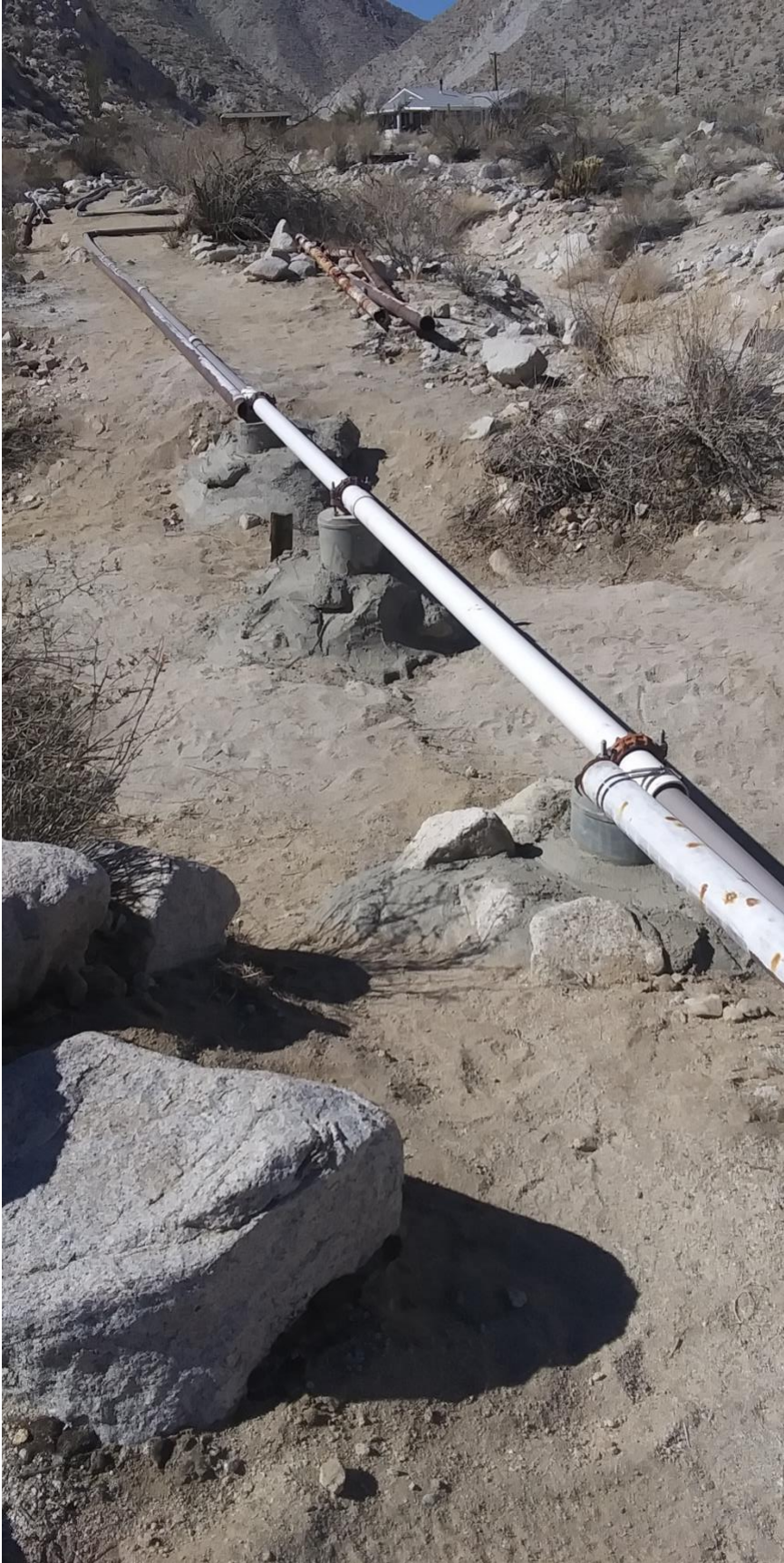
Concrete pillars used to bridge one of the washes
