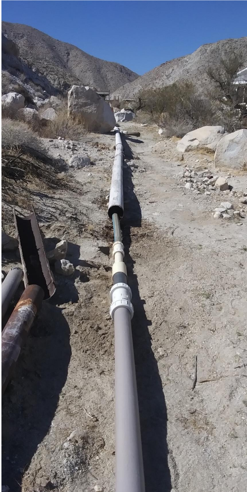
Connection to old 2-inch line
